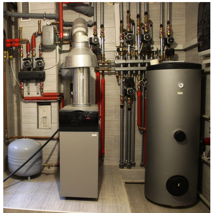
Ground source heat pump
