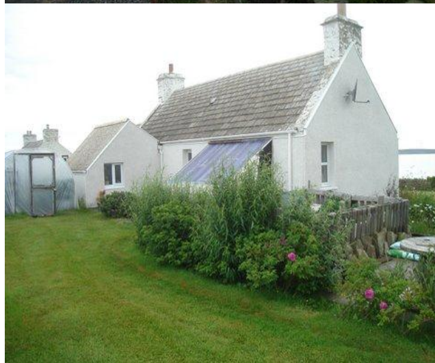
Figure 5: Orkney cottage before and after insulation
