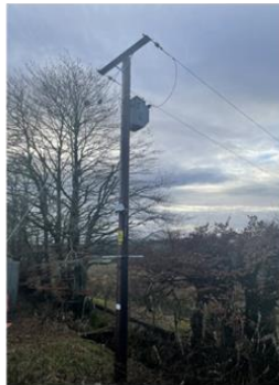
Incoming single-phase supply, from the North end of the site.
